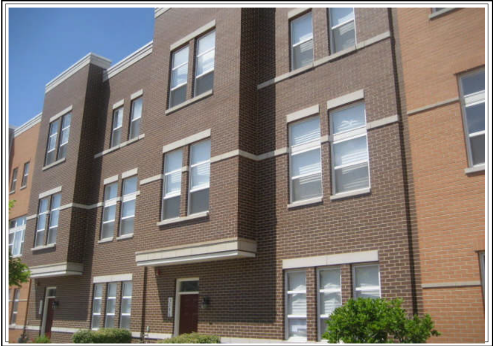
FRONT VIEW OF SUBJECT PROPERTY
